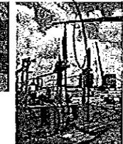
APECB with porcelain insulator, assembled horizontally on the ground before lifted & into place, Greece.
