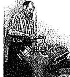
Manufacturing outdoor cable terminations for paper-insulated cables in 1962.
